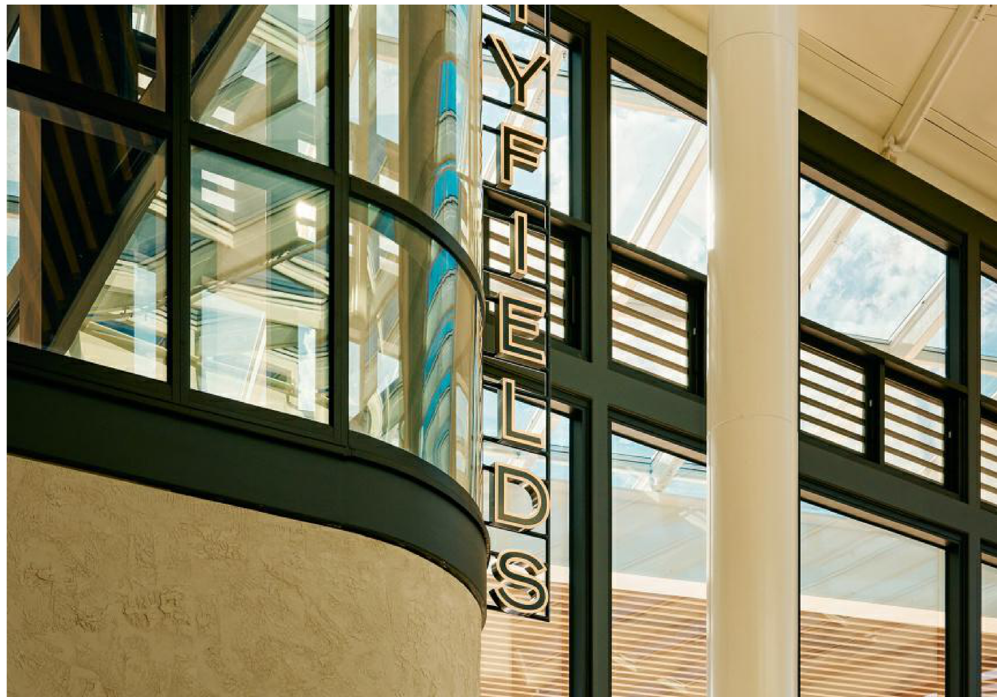
5. ALUMINIUM FRAME ON WINDOWS AND DOORS - POWDERCOAT FINISH COLORBOND - MONUMENT.
